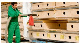
STEICOzell insulates with pure wood fibres
