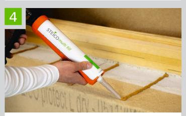
Bonding the wedge depending on insulation height with STEICO*multi fill* in adhesive beads or STEICO*secure Base* using adhesive pads,  $e \le 200 \, \text{mm}$
