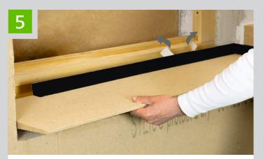
Installation of the STEICO*tri* Insulating wedge: Float fully into the adhesive with pressure. **TIP**: Fold back separating paper for easy removal
