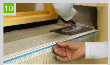
Installation: Side fabric corner angle (optional), fabric insert flat, STEICOsecure end profile FB at the leading edge
