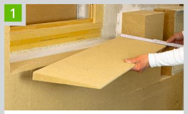
Flush cutting of the STEICO*tri* insulation wedge to the appropriate length and depth of the window opening
