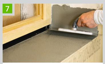
Then spread the entire wedge and the lower reveal area forward with STEICOsecure Base Guard (or similar approved render)
