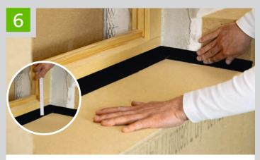
Ensure correct levelling, remove the remaining separating paper and press on the STEICO*multi tape black* all around
