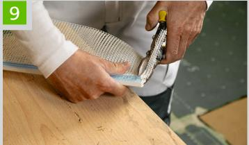
Cutting of STEICOsecure mesh 4x4, fabric corner angle, end profile FB
