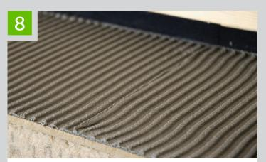
Toothing in the direction of the slope is performed with a toothed trowel 6 mm to achieve a dry film thickness of min. 4-max. 10 mm
